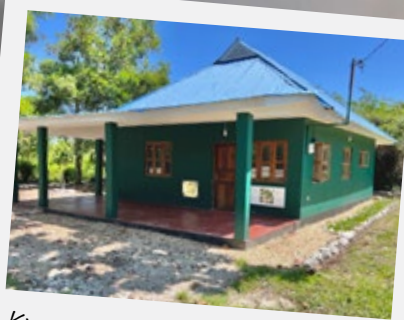
Kiwengwa - Pongwe Forest Reserve office renovated in Zanzibar.
